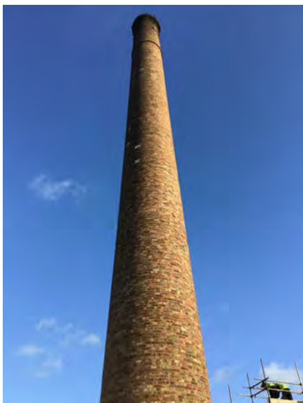
Glengall Road Chimney
