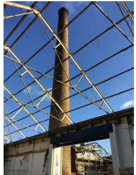
Glengall Road Chimney
