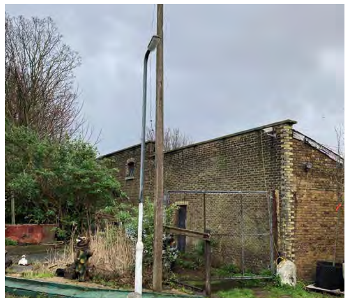
Catlin Street light column
